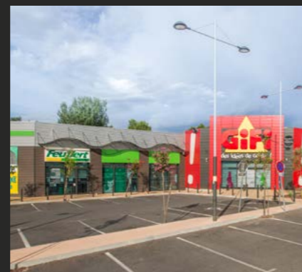
Commercial area CLAD 4 Earth France
