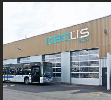
Bus station CLAD 4 & 14 Sun Contractor : STIF - Keolis
