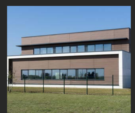
Head office CLAD 4 Heat Contractor : Veolia
