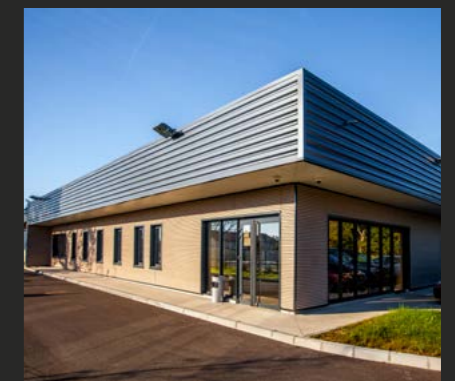
Bank branch CLAD 4 Sand Contractor : La Banque Postale
