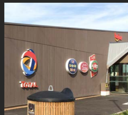
Gas station COVER 6 Earth Contractor : TOTAL
