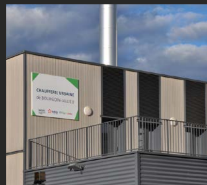
Boiler room CLAD 4 Sand & Earth Architect : Soho Atlas
